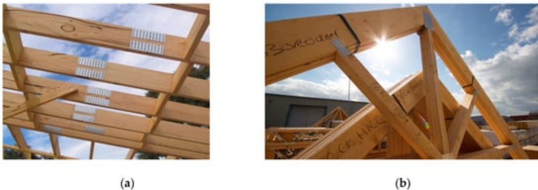
Figure 8. Examples of connections made with nail-plates [24] [25] .
